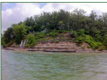
Picnic Island Erosion Control Project Completed– Summer 2013
