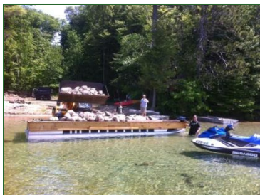
Picnic Island Erosion Control Project Under Construction – Summer 2013
